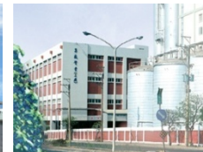
DTY Plant III 1997
